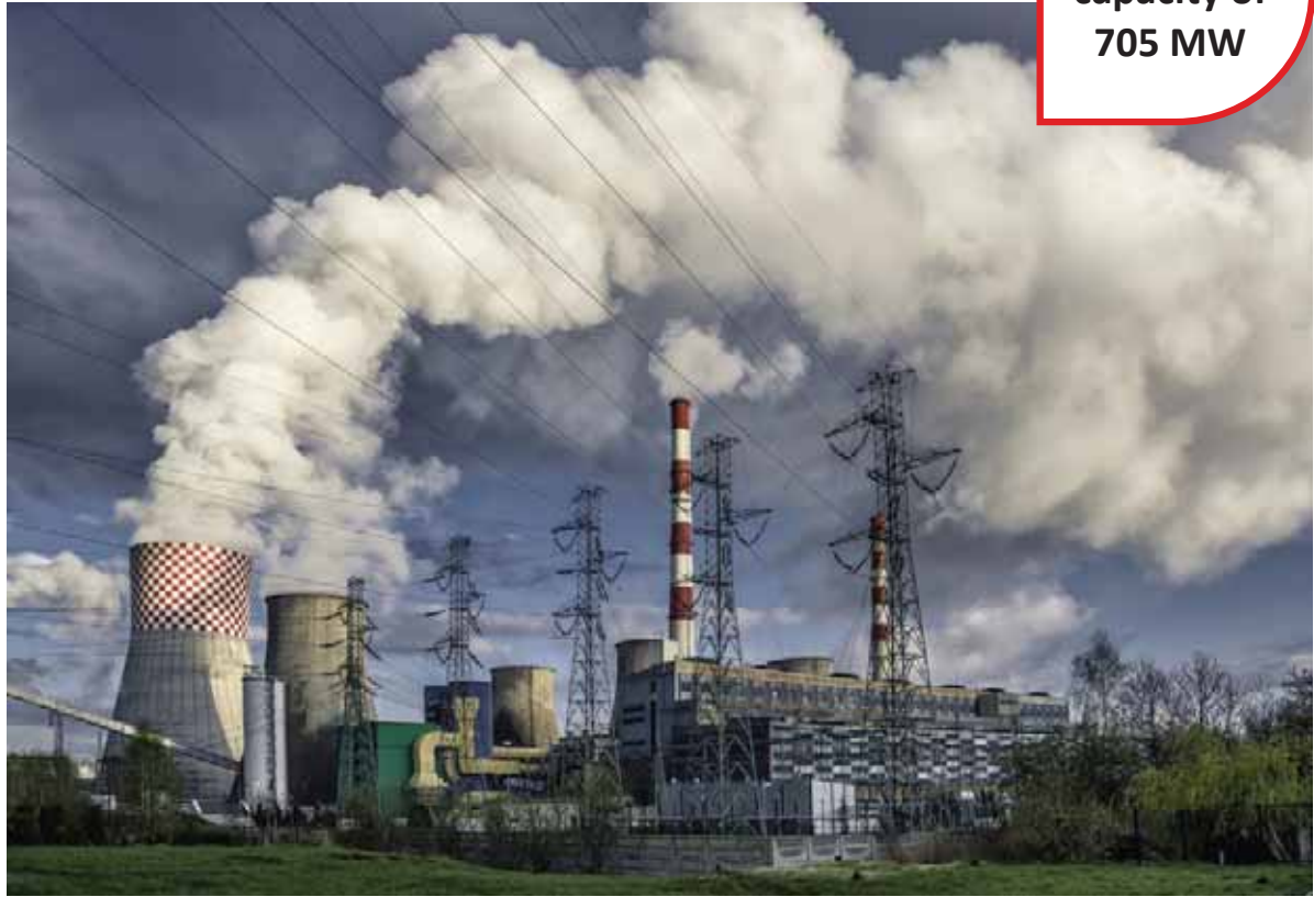
Delhi's biggest power generator in Badarpur was shut down in October 2018
